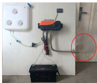
Excessive pump oil produces white smoke
